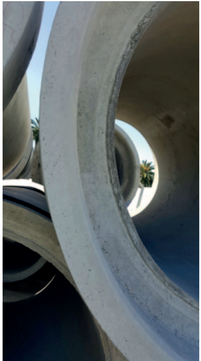
Pipes with sacrificial layer
